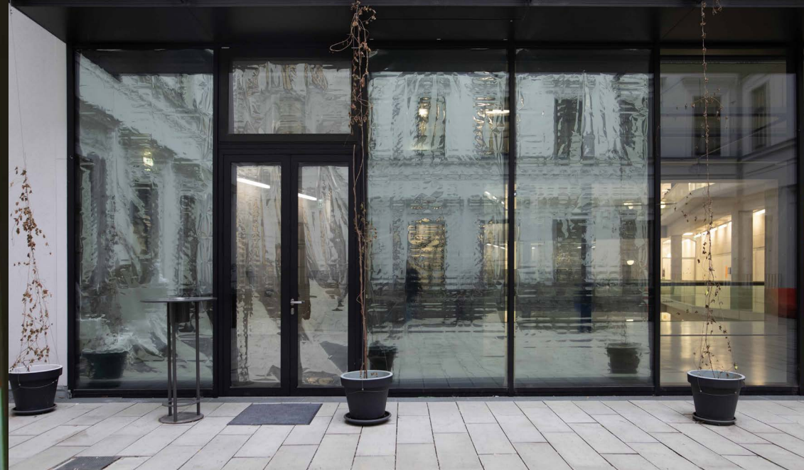
The spy film used in police stations was applied to a large part of the window front to create darkness in the interior. Furthermore, it is not possible to see through the reflective film from the outside during the day, but it is possible to see through it from the inside. In the evening, the effect is reversed and visitors see their own reflection inside the room, while they can be observed from outside.
